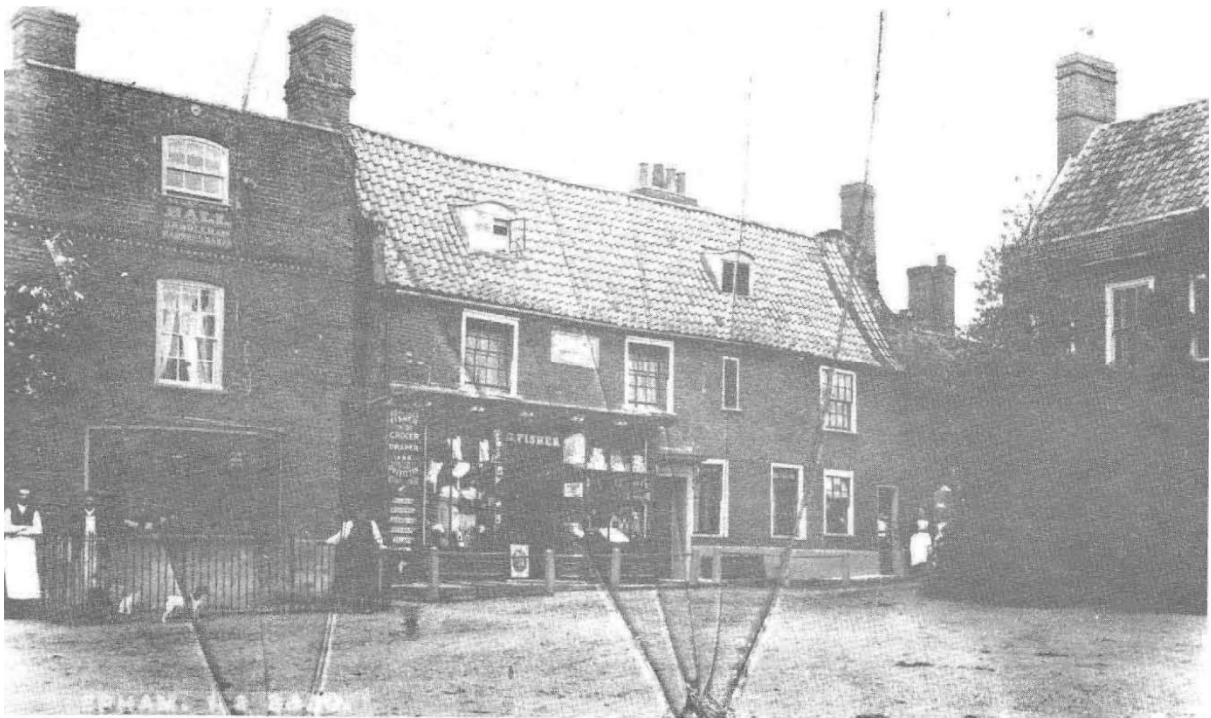
Probably taken in the 1890s – showing the original roof line of Hall's shop (the saddler and harness maker)
