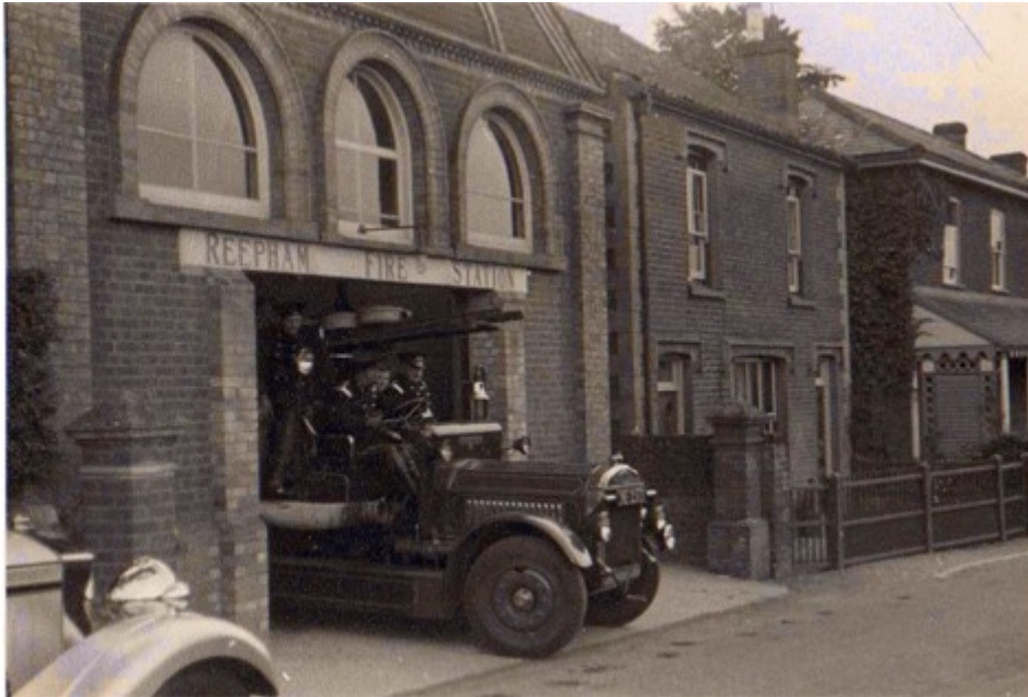
Reepham Fire Station on Dereham Road, possibly late 1930s.
