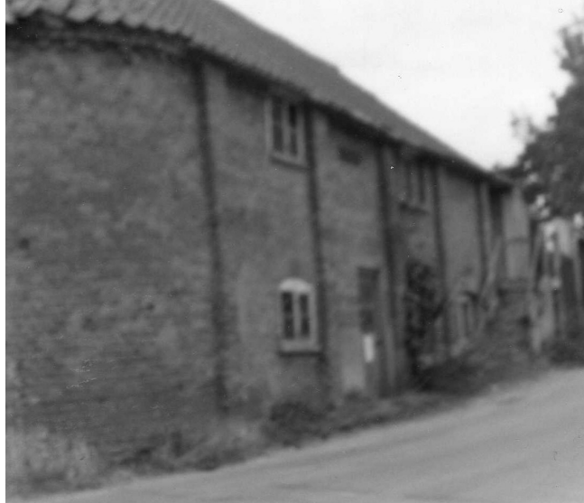
The Maltings looking across Ollands Road from Malthouse Yard (the wall is not quite so tall now, the windows are bricked up and there's a big blue tin gate where the outside stairs were)
