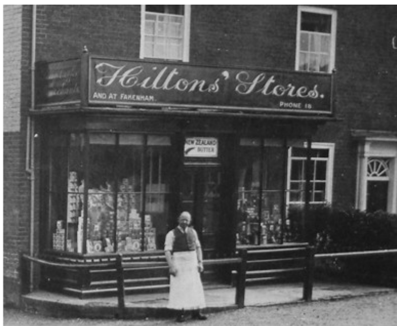
Hiltons' Stores in Reepham Market Place (now the police station, in 2017)
