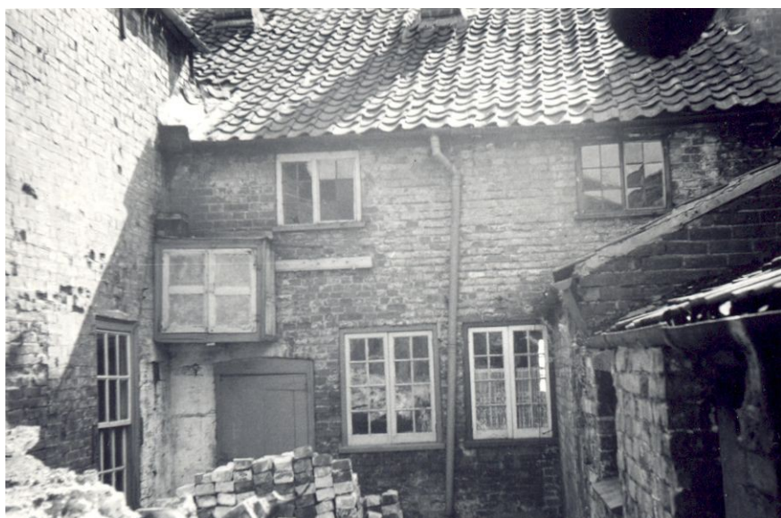
The back of the older part of the house showing the meat safe, reached by climbing a ladder.
