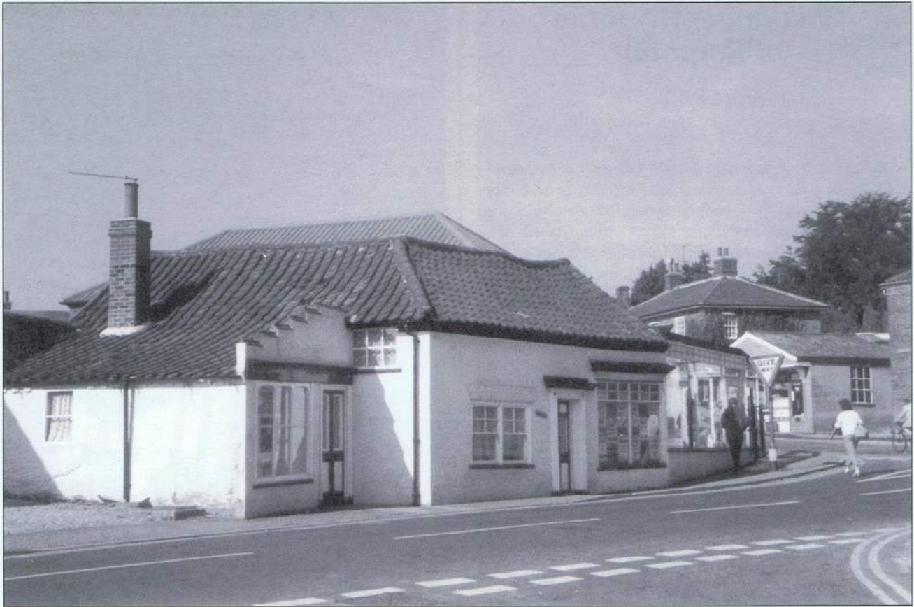
This was the site of the shop formerly run by Mr and Mrs Ron Gibbs at Towns End Corner. It has now been pulled down and replaced by the new development containing the hairdresser, DIY shop and electrical shop.
