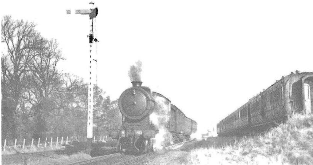
D 16/3 No. 62562: Before the passenger traffic declined in the 1950s the 10.41 am from Melton to Norwich leaves Whitwell in February 1949.
