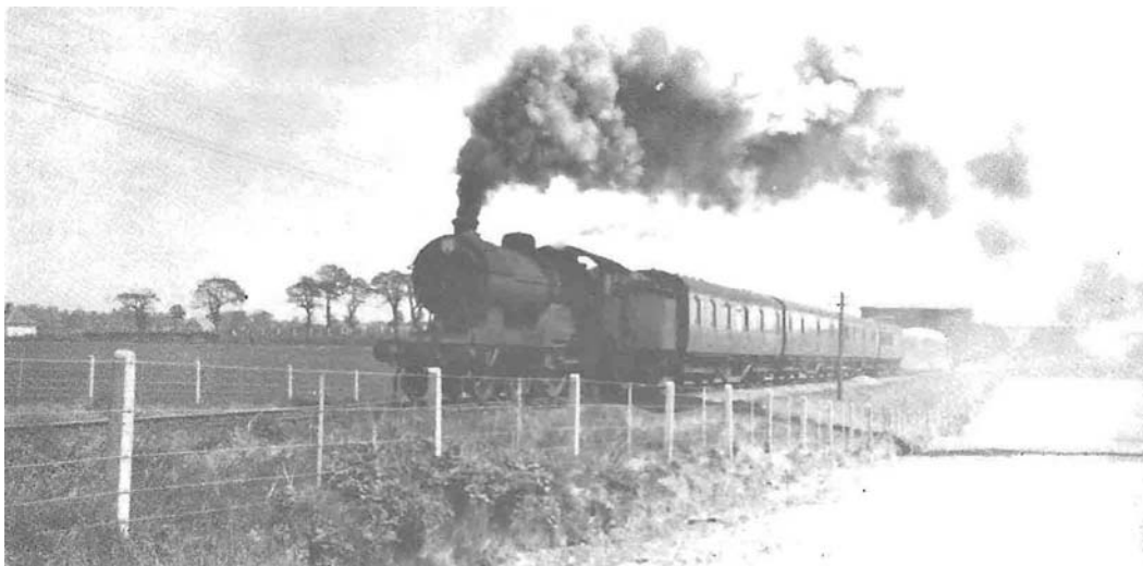
D 16/3 No. 62533: Hackford Bridge was removed a few years ago; this shows a full head of steam as the train heads from the bridge towards Themelthorpe in May 1957.
