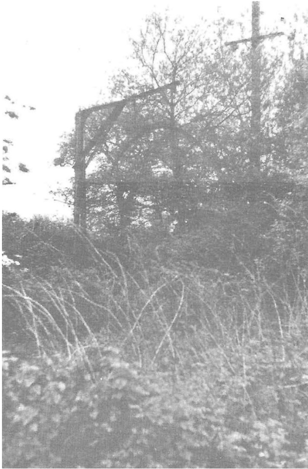
The loading gauge, unused now for 30 years and nearly smothered by nature's unchecked growth.
