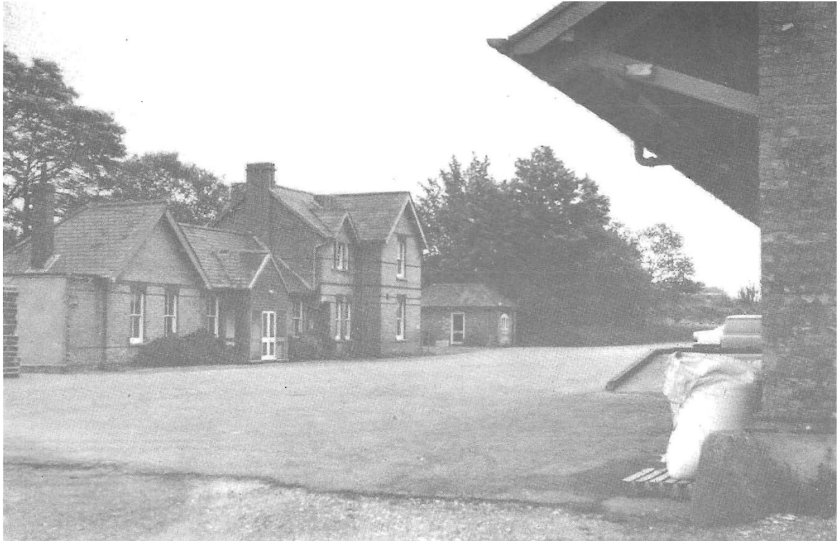
A present-day view of the station buildings. The parcel building is the small separate unit to the right. The two-storey part of the building was the station master's house.
