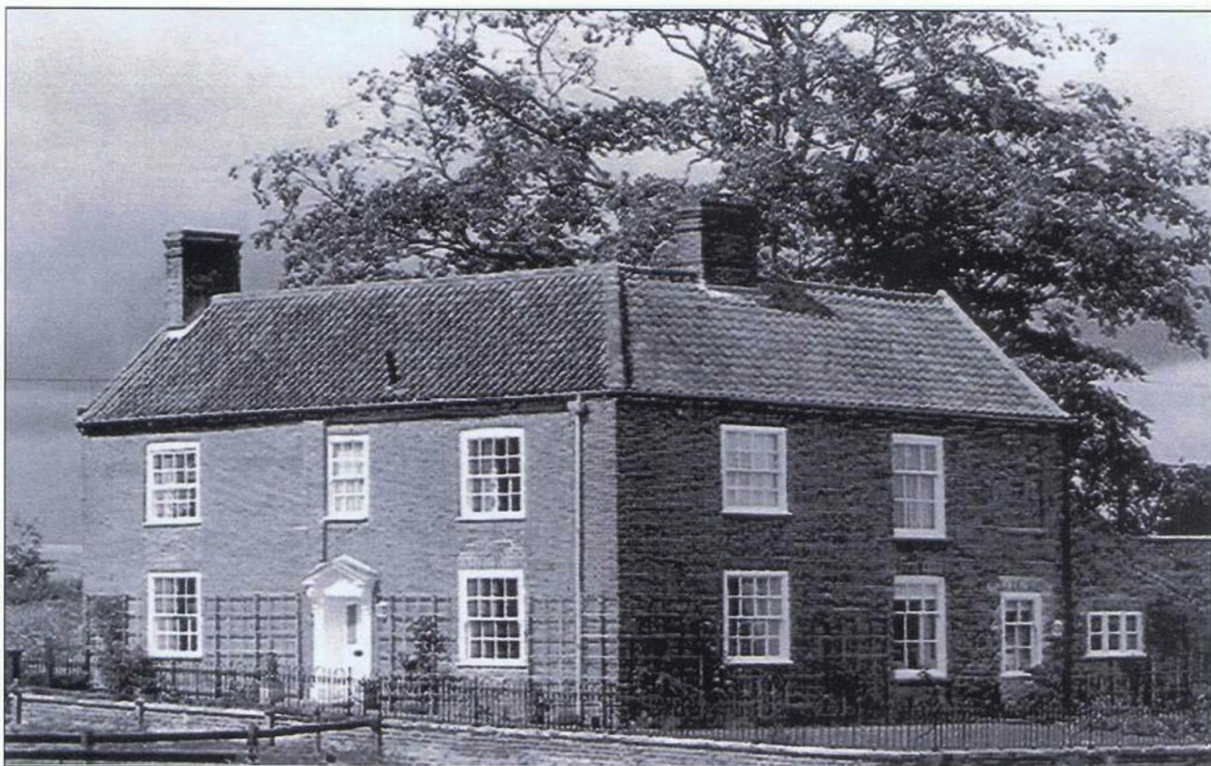
Pettywell Place now lived in by Howard and Margaret Blandford-Baker was formerly owned by the Eglington family. In 1846 it was owned by John Sewell but occupied by Margaret Rodham.
